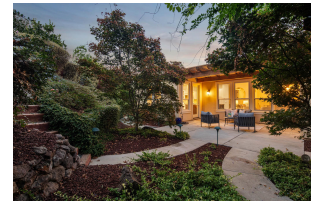
Back Of Structure
